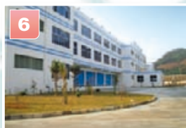
6 Huang Jiang Plant
